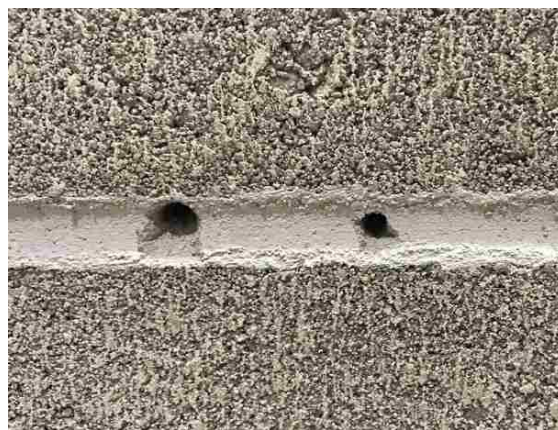
Figure 3-9: Original Helix Hole and Secondary Pilot Hole
